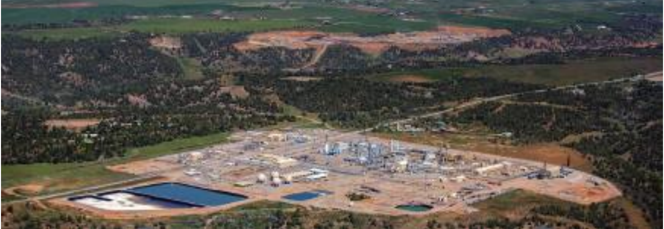
Hilcorp Energy Ignacio Gas Plant Waste Heat to Power Project – Durango, Colorado
