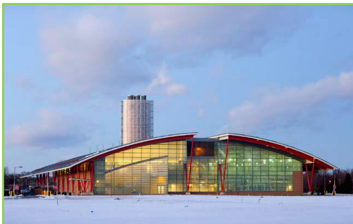
UMass Amherst's central heating plant
