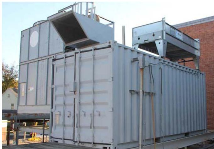
The 335kW CHP systems is housed in two separate containers. The first to be installed was the 250kW AMERIGEN8250, followed by the 85kW AMERIGEN8085
