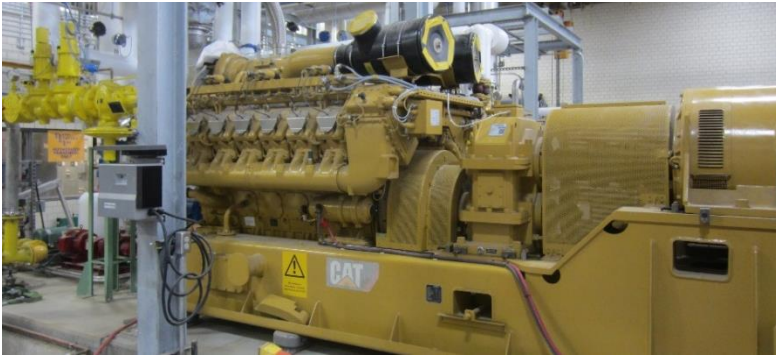
1.2 MW CAT Engine (CAT CG170-12) Photo Courtesy of City of Springfield
