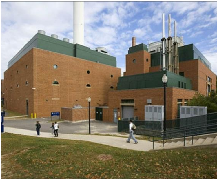
University of Connecticut's Central Utility Plant (CUP)
