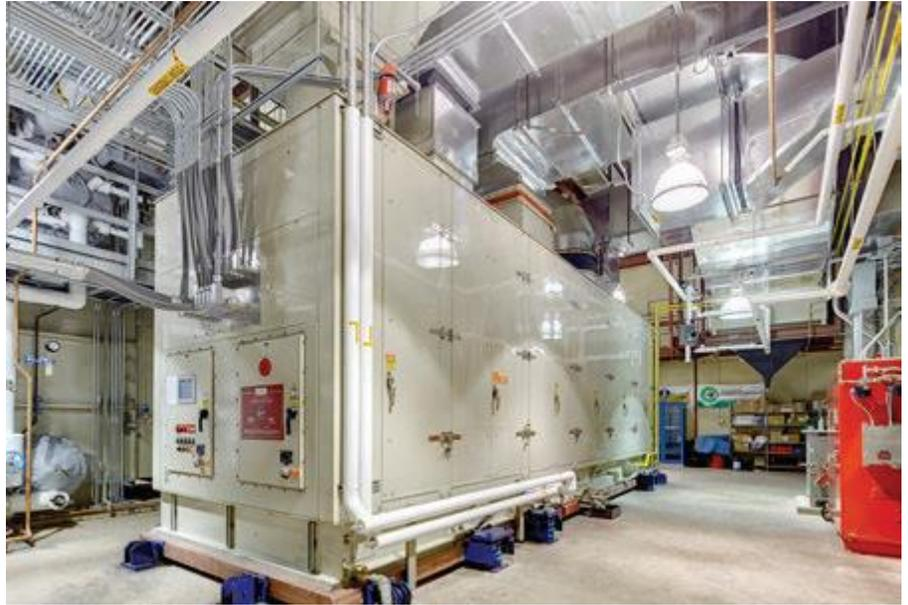
Location of a viable site for the CHP plant within the hospital was a challenge. However, the project team was able to locate and utilize space over a loading dock and under an overhang of the existing building. Fitting a 4.6 MW plant over a loading dock serves as a testament to the versatility and compact footprint of a well-designed CHP system.
