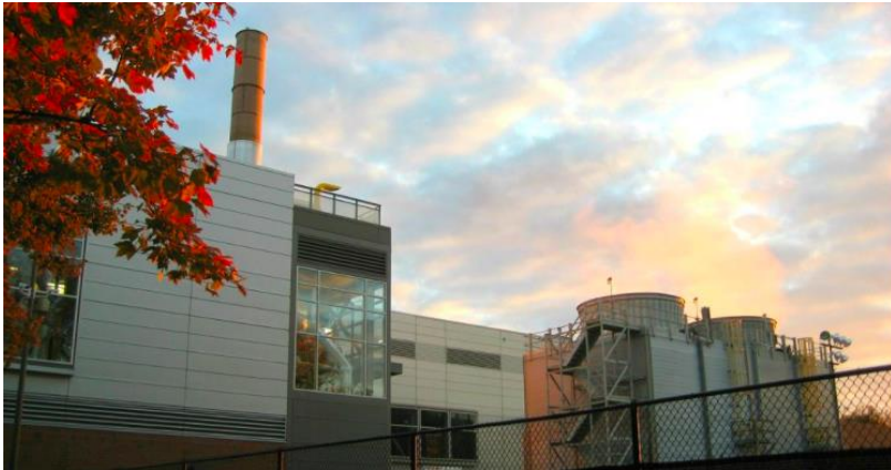
NC State's Cates Utility Plant houses 11 MW of the 17.5 MW total Combined Heat and Power now on campus.
