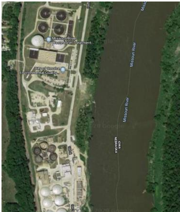
An Aerial View of the Missouri River Resource Recovery Facility (Source: Google Maps)
